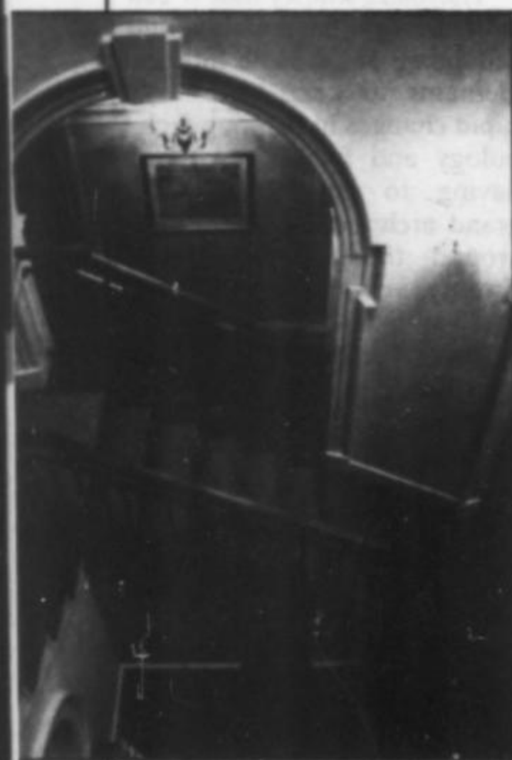
Top, general view of exterior from Agricultural Hall Plain; above, main stair - designed to be hard wearing as well as elegant; centre, skilful addition at rear of building - delivery area.
